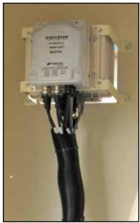
Fig 66 - Weigh Scale junction box
